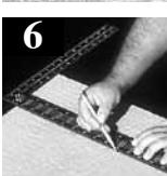
6. Using a square, draw a centerline perpendicular to the outside edge of the platform.
