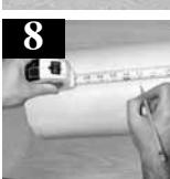
8. Use a wood rasp to level top of column shaft. Measure from the top of the column to the proper length and make a series of marks around the column shaft.
