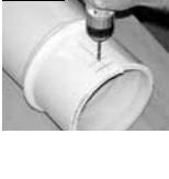
18. \* Slide the cap up to the beam and push up until secure. Screws may be used to secure the cap to the beam and the base to the platform. (When using screws, first drill pilot holes and fill with putty to cover screw heads.)
