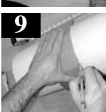
9. Using a piece of cardboard as a guide, draw a line all the way around the column.
