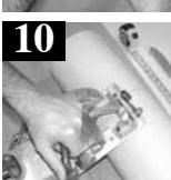
10. Cut the column using an abrasive circular saw.
