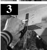
3. Determine the top centerline and mark it on the beam.
