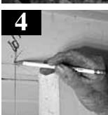
4. Hang a plumb bob from the top centerline to determine the bottom centerline.
