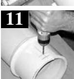
11. Mark and drill clearance holes on the top and bottom of the column to accommodate bolts for the 1-3/8" L-brackets (L-brackets sold separately).
