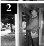
2. Using a jack and post, jack up the beam only enough to remove the existing post, no more than  $\frac{1}{4}$ ".
